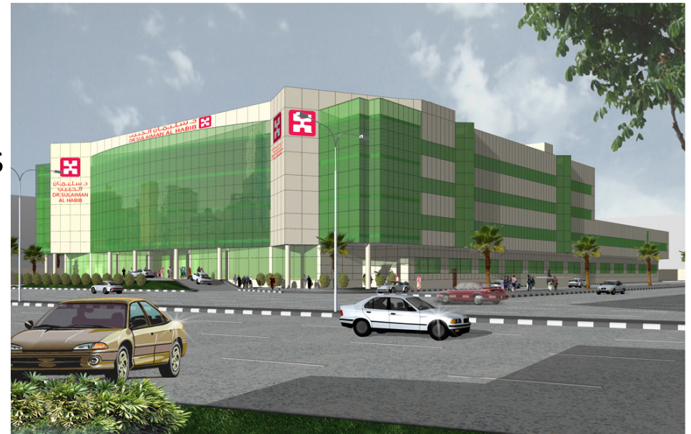
AL RAYED HOSPITAL TAKASSUSI ROAD - RIYADH
